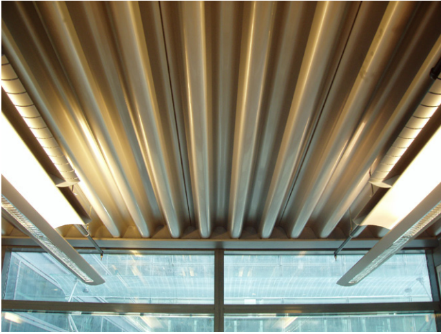
Fig. 6. Exposed stainless steel floor decking at the Luxembourg Chamber of Commerce.
